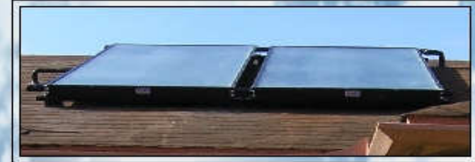
Solar Panels Installed
